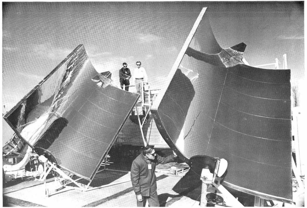
PARABOLIC TROUGH REFLECTORS measuring 9x12 feet, part of Sandia's solar energy research program, were recently installed in the northwest corner of Area I. The giant mirrors are made of fiberglass and polyester with a lining of aluminum reflector sheet. Not installed yet, the "plumbing" will include receiver tubes at the foci of the reflectors. A storage tank with associated instrumentation, pumps and
